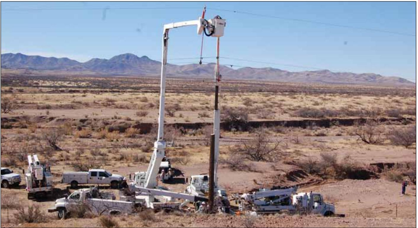
*Setting a pole and safely electrifying a line bearing 69,000 volts requires the right equipment and reliable vehicles. This team of SSVEC journeyman linemen depend on a well-maintained fleet.*
